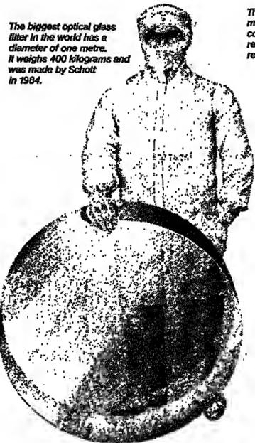
The biggest optical glass filter in the world has a diameter of one metre. It weighs 400 kilograms and was made by Schott in 1984.
